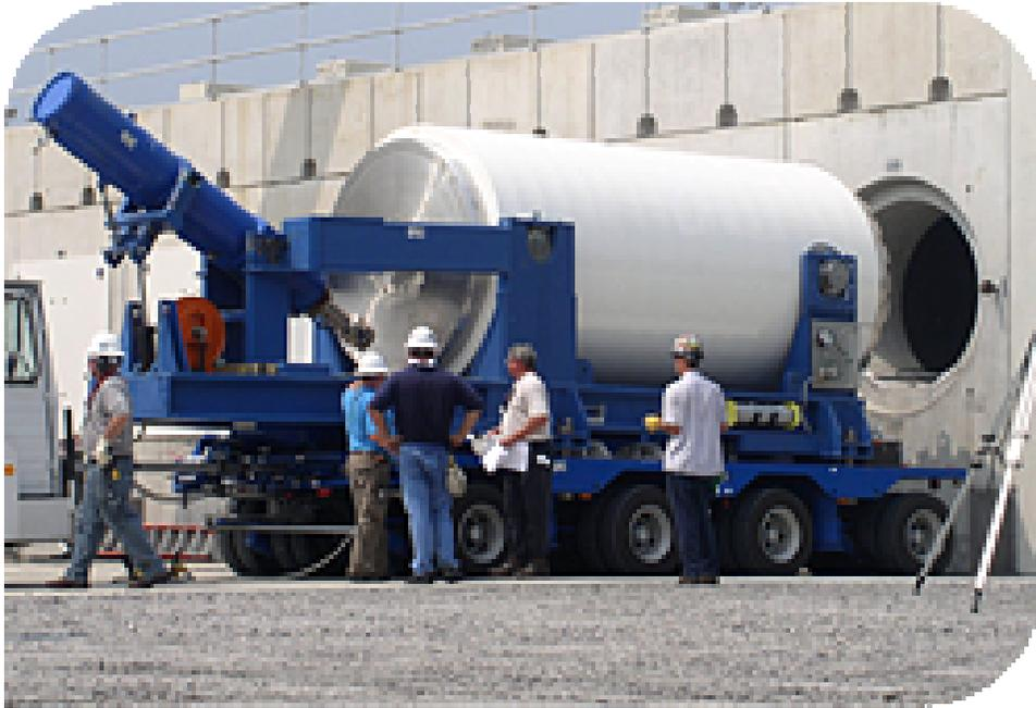
**Fig. 3. NUHOMS canister fits inside a concrete overpack.**
